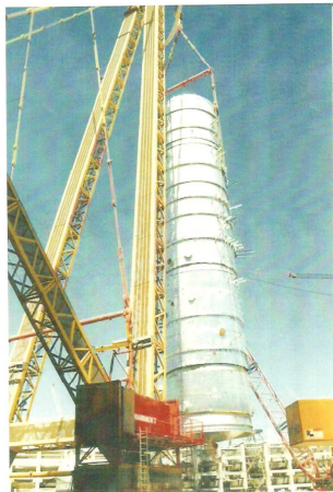
UNIT : FCCU, RIL SEZ EQUIPMENT : FCC ERECTOR WEIGHT : 1000 MT
